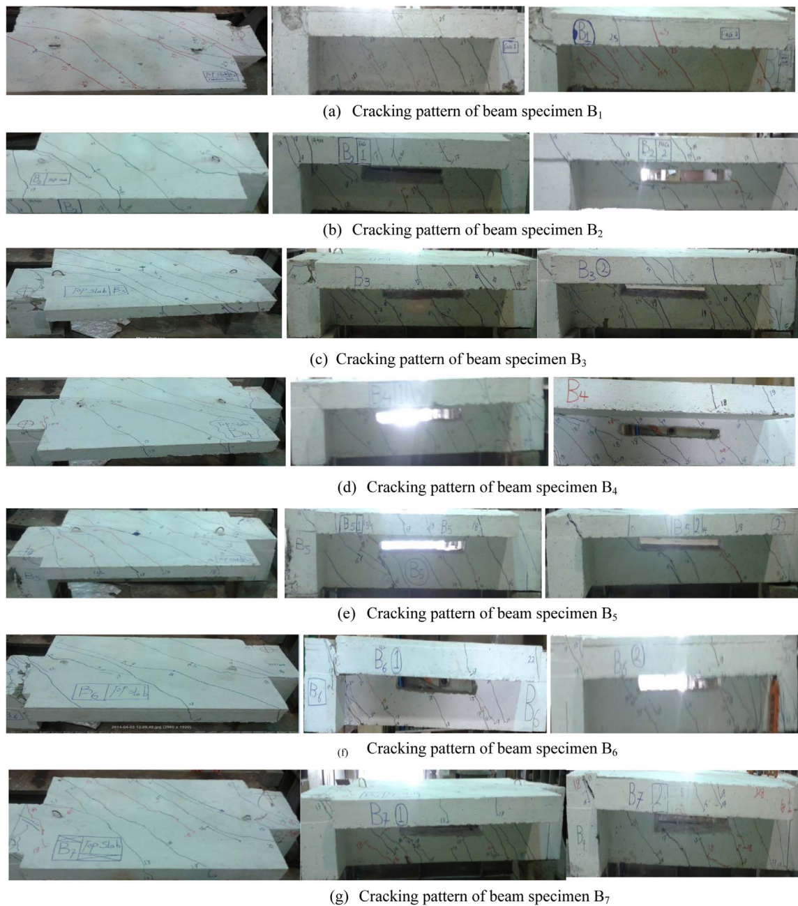
Fig. 4. Cracking patterns of the tested specimens in horizontal and vertical faces.
